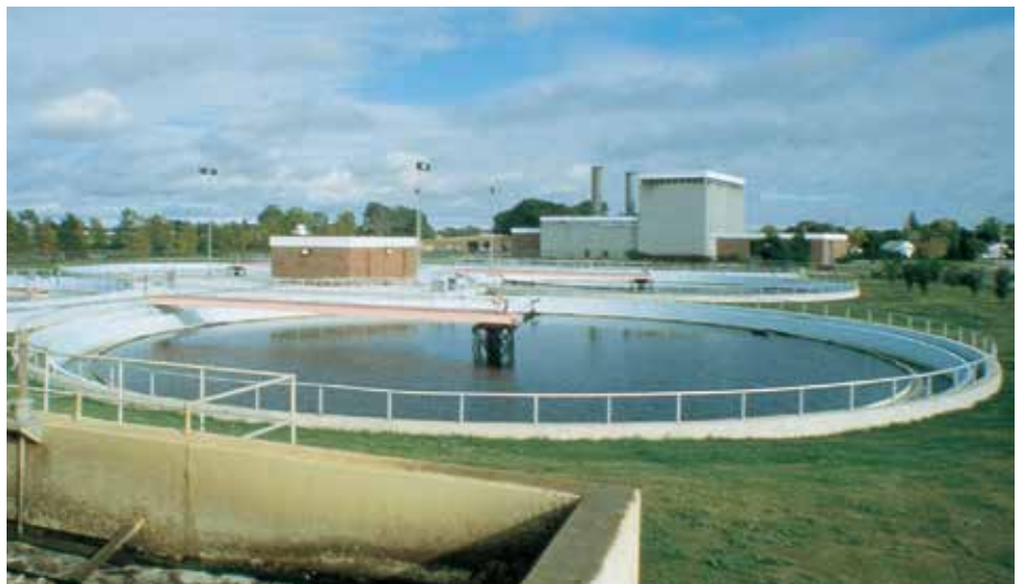
Four 120-foot diameter Rim-Flo® Clarifier tanks operate at 700 GPD per square foot of overflow in this installation. Effluent quality is 3 to 7 ppm BOD and SS.
