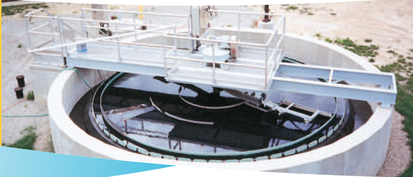
35' diameter Full Bridge Clarifier
