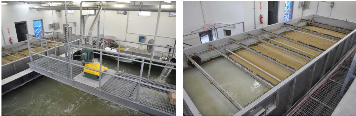
Figure 4. Full-Scale Flash Mix Tank and Tertiary DAF
