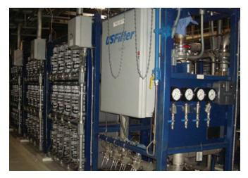
**Figure 1** 6,750 gpm (1500 m<sup>3</sup>/h) boiler feed water CEDI system (1 of 10 skids). USFilter is now part of Evoqua Water Technologies.
